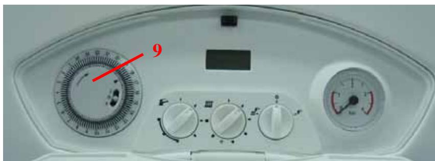
**(9)** A time clock allowing the automatic switching 'On' and 'Off' of the central heating is fitted as standard.
