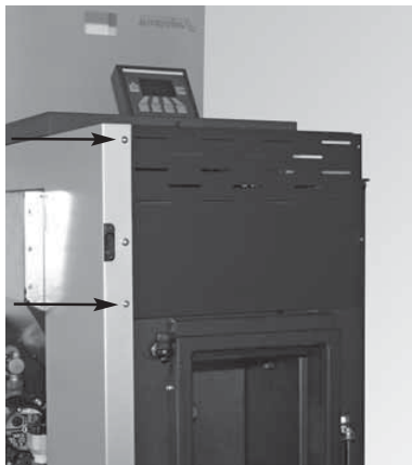
Fig. 30 Screwing the front cover plate on at the front at 2 points
