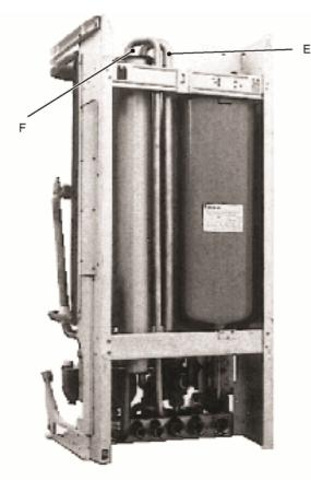
6 Remove the bracket that holds the heat exchanger to the frame (top plug side) by unscrewing the screw that fastens it to the frame
