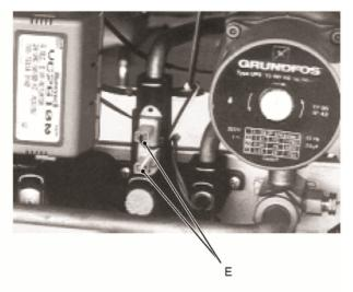
Measure the electrical resistance at the leads of the sensor. Without water being drawn, the contact must be open. By opening a hot water cock the contact must close (electrical resistance zero  $\Omega$ ).
