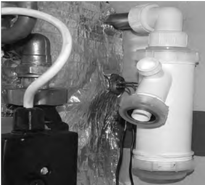
Figure 6-2: Condensate trap
