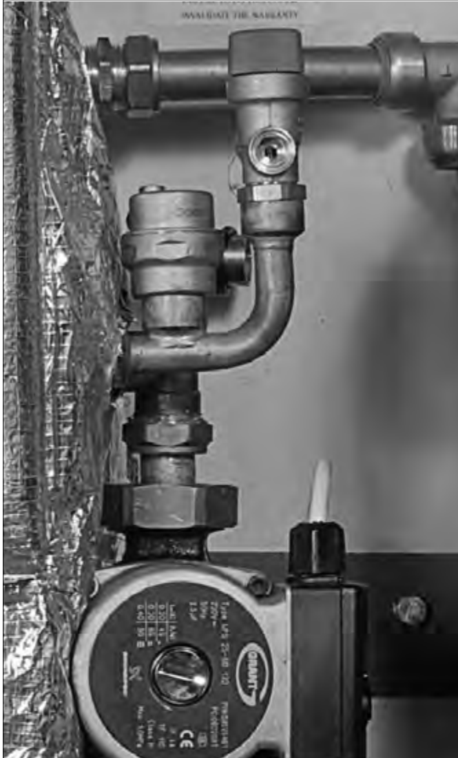
Figure 4-3: Removing flow and return pipe
