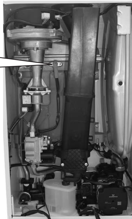
Flame Detection Electrode
