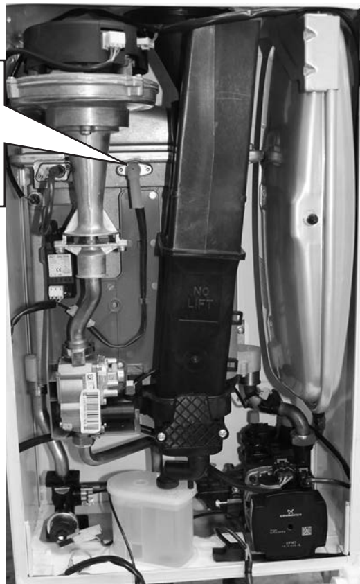
Flame Detection Electrode
