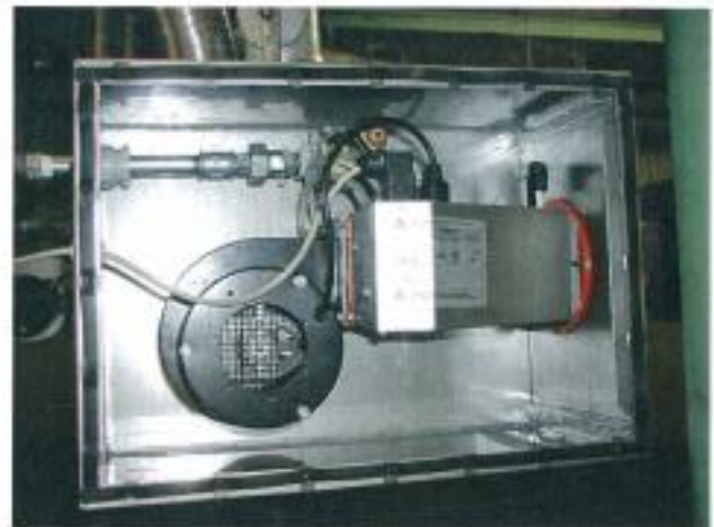
Fig. 31: Burner unit in water protection cover (without cover plate)
